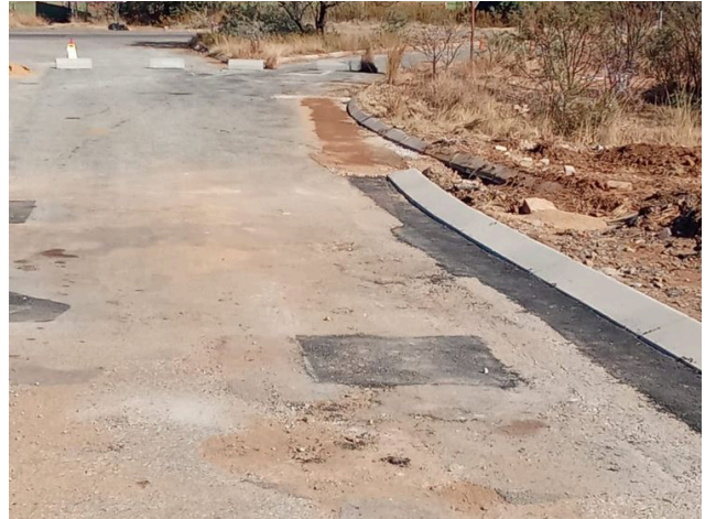
THE ROUTE CLOSED AT THE FAILED CROSSING • NEW KERB AND CHANNEL ALONG THE APPROACH
