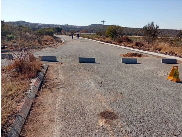
THE ROUTE CLOSED AT THE FAILED CROSSING • NEW KERB AND CHANNEL ALONG THE APPROACH
